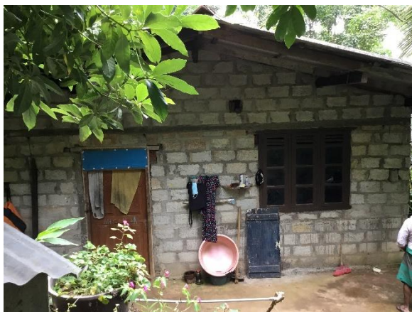
High Risk houses located downslope
