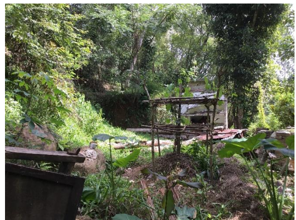
Damaged house from landslide incident
